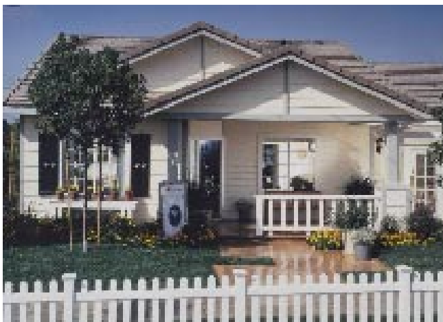
Example of residence that demonstrates a successful relationship with sidewalk and street
